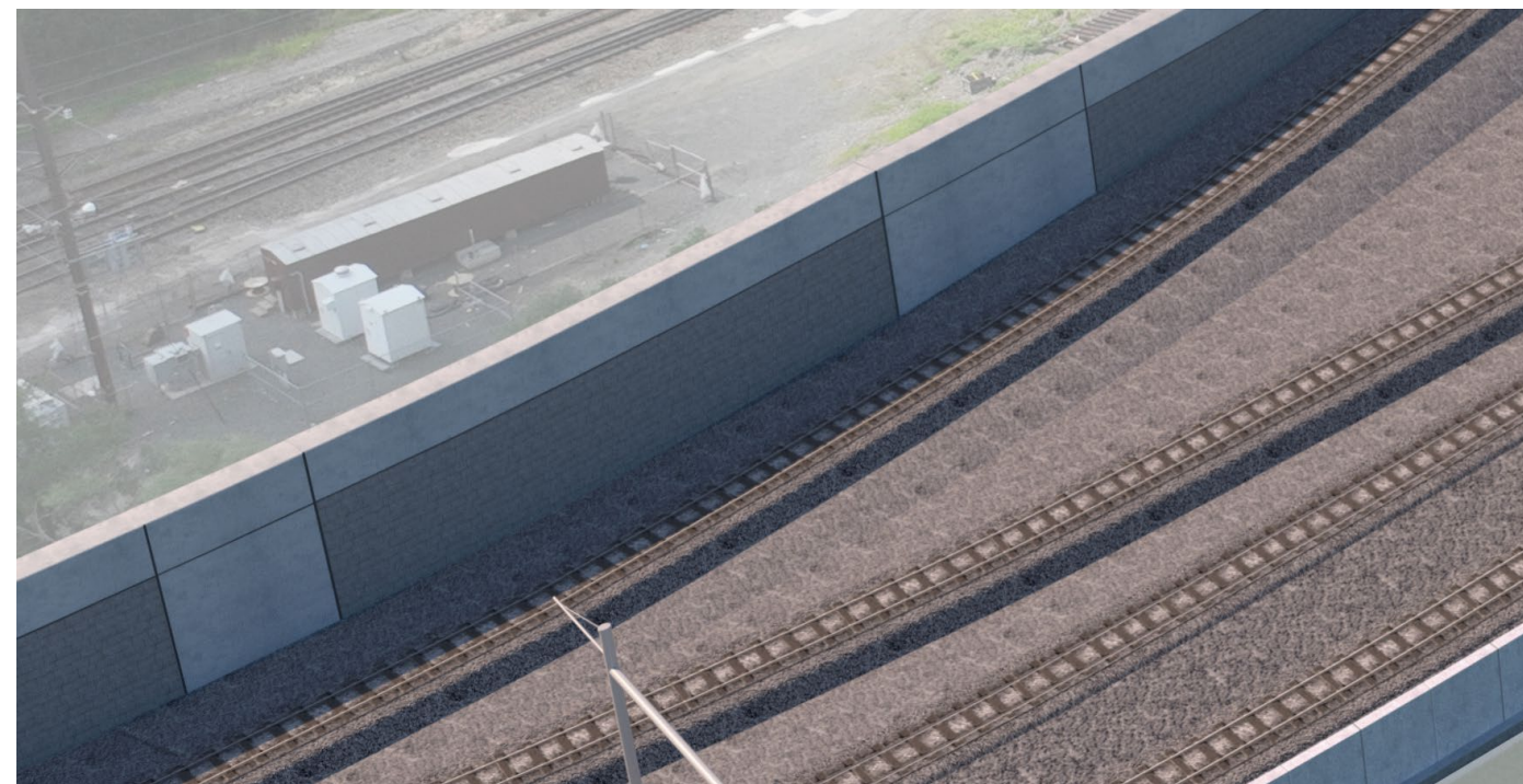
New retaining walls aesthetically blend the rail line's historic use of stone and concrete.
