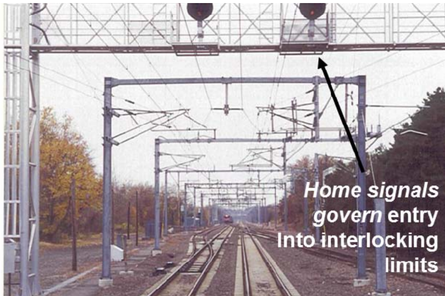
“A” Interlocking in New York Penn – signals displaying green over red indicate “Clear,” and show a route has been lined through the interlocking
