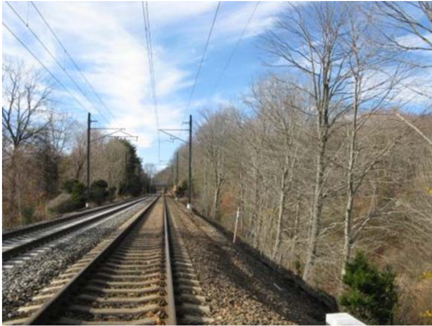
Catenary north of New Haven uses a 25,000 volt system dating from the late 1990s.
