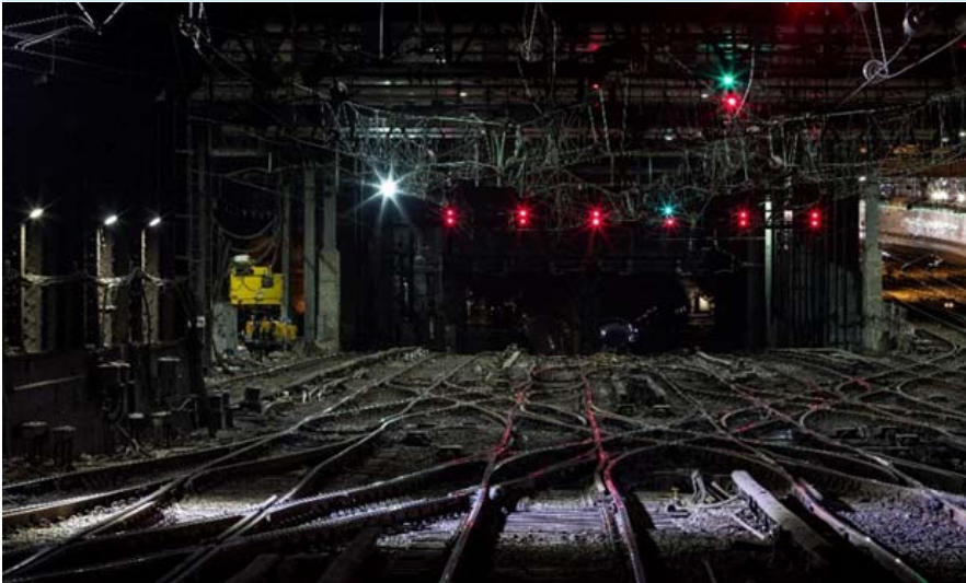
“A” Interlocking in New York Penn – signals displaying green over red indicate “Clear,” and show a route has been lined through the interlocking
